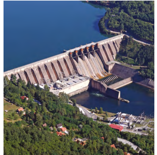
Power Generation & Utilities
